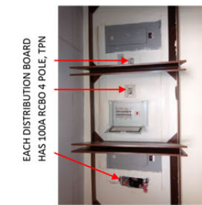
FIG.16 – 3NOS DISTRIBUTION BOARDS (First floor) same arrangement as ground floor
