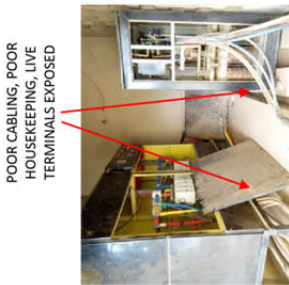
FIG.9 – VOLTAGE STABILIZER, NOT FUNCTIONAL. (Generator area )
