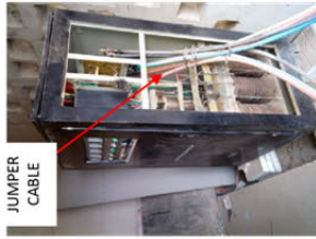
FIG.10 – CHANGEOVER PANEL. EXPOSED LIVE BUSBARS. NO INGRESS PROTECTION. (Generator area)
