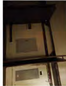
FIG. 16 - 3NOS DISTRIBUTION BOARDS (First floor) same arrangement as ground floor
