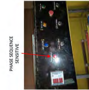
FIG. 11 - CHANGEOVER PANEL. WITH AUTO AND MANUAL SWITCHING PROVISIONS. (Generator area)
