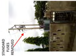
FIG. 13 - 500KVA TRANSFORMER, FEEDER PILLAR, HT POLE (Transformer area)
