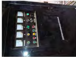
FIG. 12 - VOLTAGE STABILIZER DISPLAY METERING AND INDICATORS. NOT FUNCTIONAL (Generator area)
