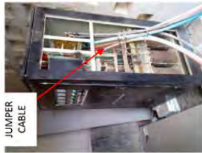
FIG. 9 - VOLTAGE STABILIZER. NOT FUNCTIONAL. (Generator area)
