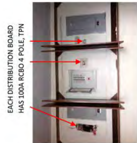
FIG. 15 - 3NOS DISTRIBUTION BOARDS (Ground floor)
