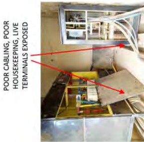
FIG. 8 - VOLTAGE STABILIZER AND CHANGEOVER SWITCH. (Generator area)
