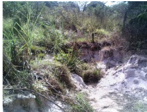
Photography 6: Soil in slope
