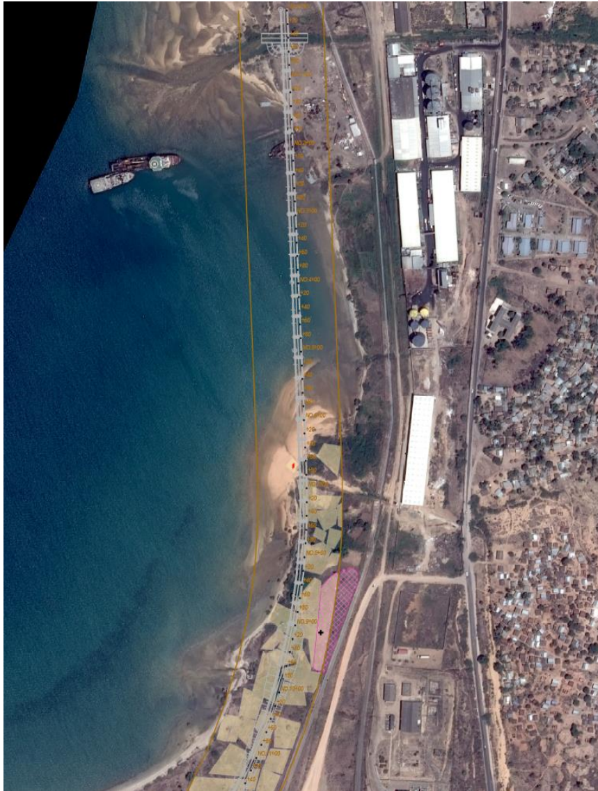
Figure 39 : Location of the floating plant and the power line tower
