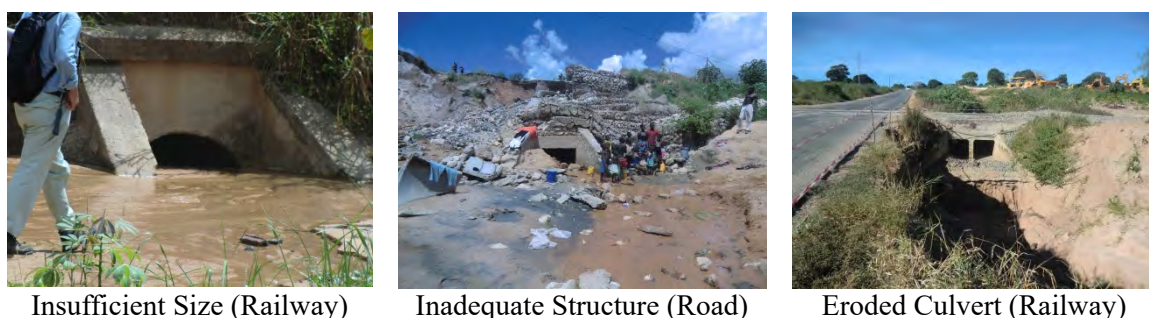
Figure 8.4.1 Existing Drainage Structures in Nacala
