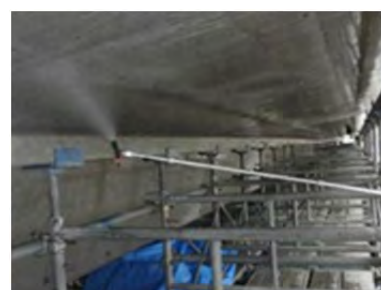
Anti-Corrosion Coating on Concrete Structure
