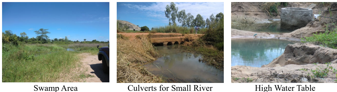
Figure 8.3 Swamp Area and Existing Drainage Facilities in Nampula
