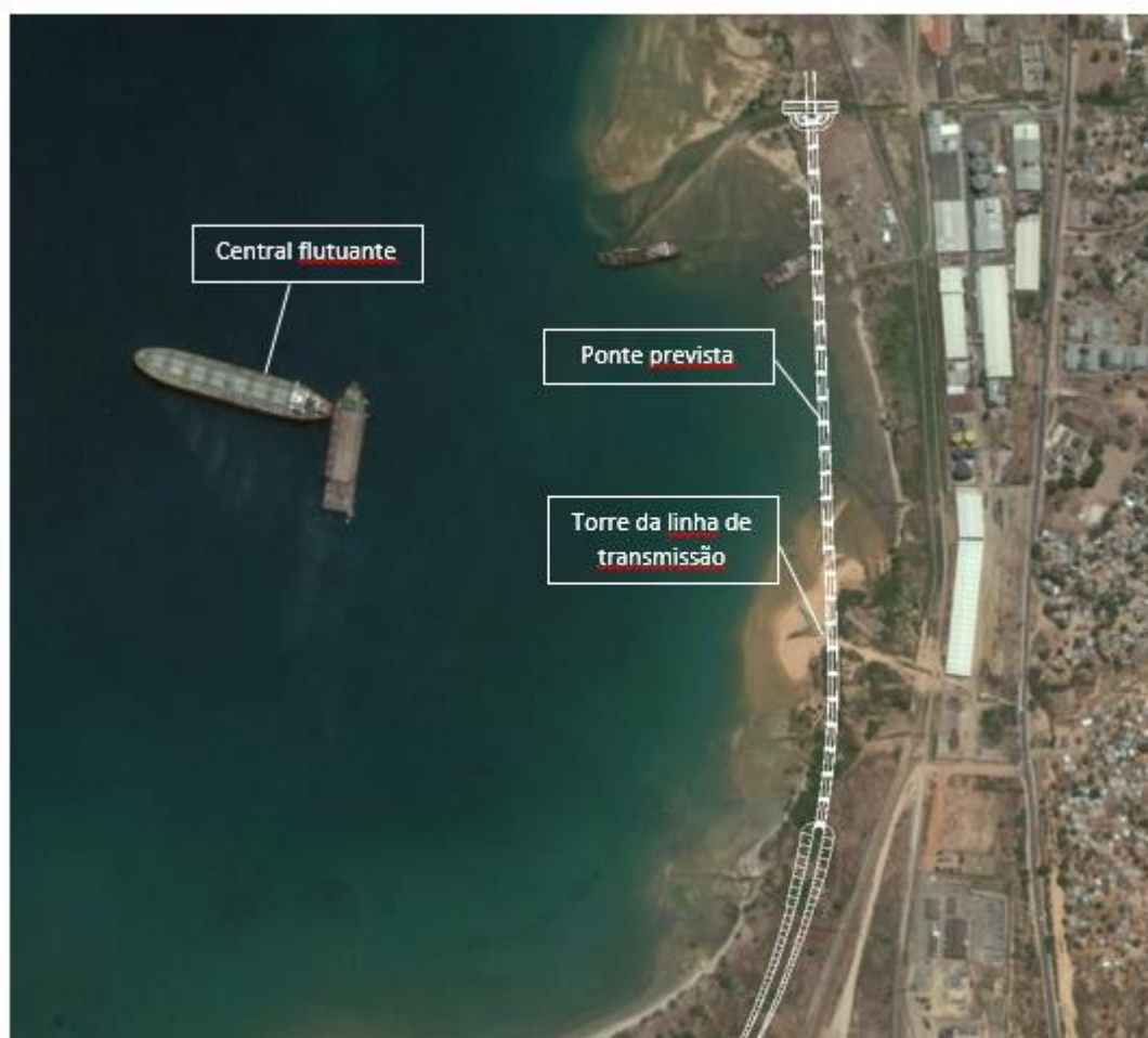
Figure 37 : Location of the floating plant and the power line tower
