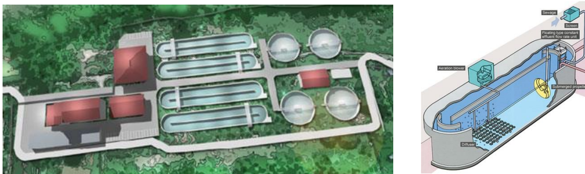
Figure 4.3-2 Kandy Sewage Treatment Plant (14,000 m 3 /day, OD Process with Nitrogen removal)
