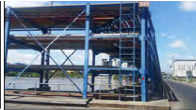
CPO Pipeline (31 units)
