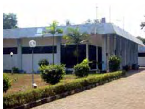
A Switching Center Built by the Extension and Improvement of Telecommunications Networks in Expanded Jakarta Areas
