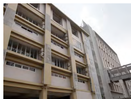
Teaching hospital under the construction at the University of Indonesia
