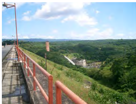
Hydropower Waterway Facilities Provided Downstream of Karangates Multi-Purpose Dam
