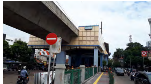
Elevated Juanda Station
