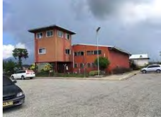
Photo 53 Fire Station View from Landside
