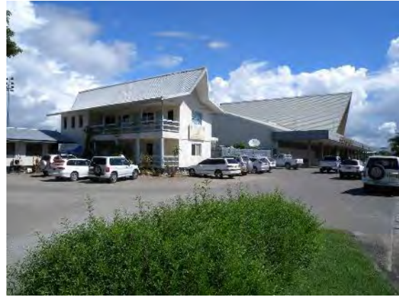
Photograph 2 International Building View from access road
