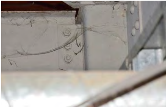
Photo 22 Condition of the Structure of backside of the Ceiling (1)
