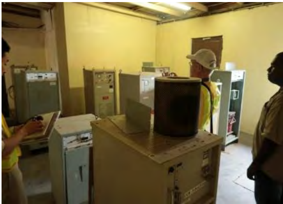
Photo 62 Inside CCR Building
