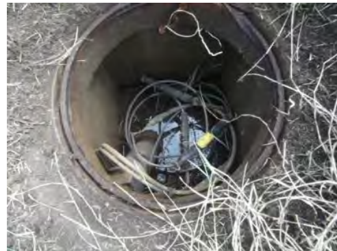
Photo 5 Hand Hole of TEDL with Cover
