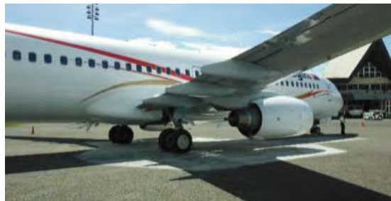
Photo 1 Concrete Pavement on the Parking Spot
