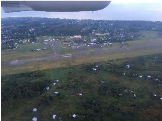
Photograph 1 Aerial view of Honiara Airport Runway in front and international building far side
