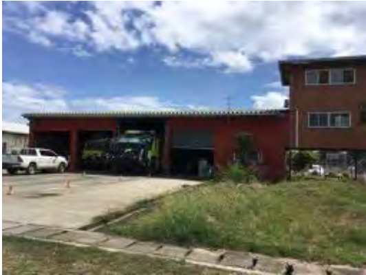
Photo 52 Fire Station View from Airside
