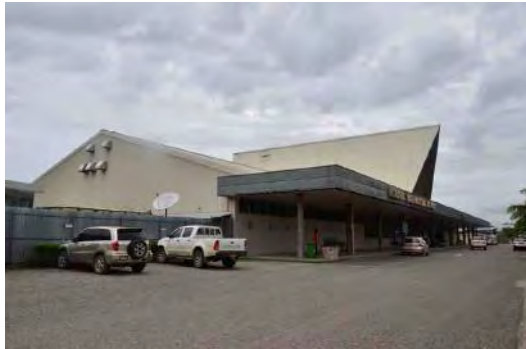
Photo 13 International Passenger Building
