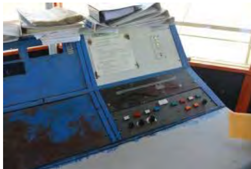
Photo 10 AFL Console in the Control Tower
