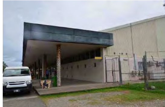
Photo 14 Exterior Finishing of International Passenger Building
