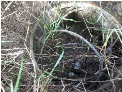
Photo 4 Hand Hole of TEDL without Cover
