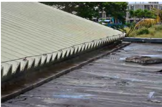
Photo 15 Asphalt Waterproofing (1)
