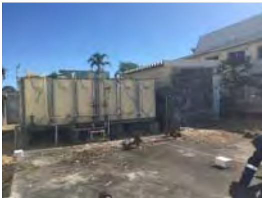
Photo 30 Water Supply System
