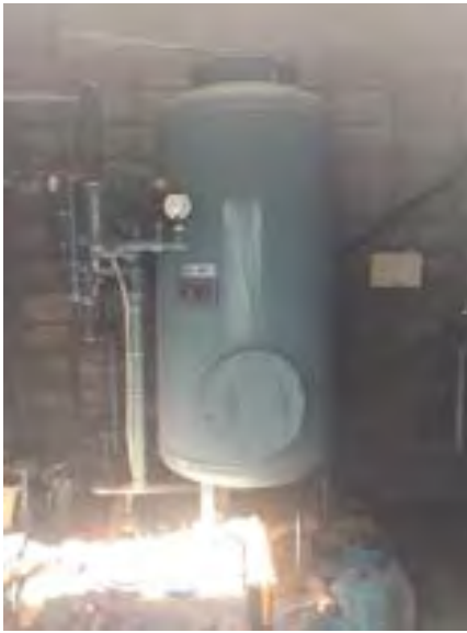
Photo 34 Pump Filter Unit
