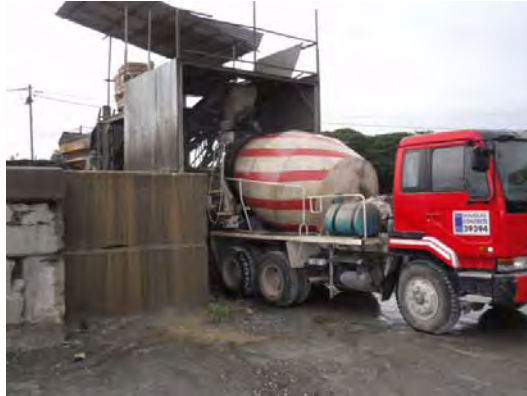
Photo 65 Concrete plant of Douglass Concrete
