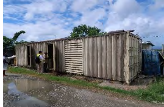
Photo 61 Container Room of Generator
