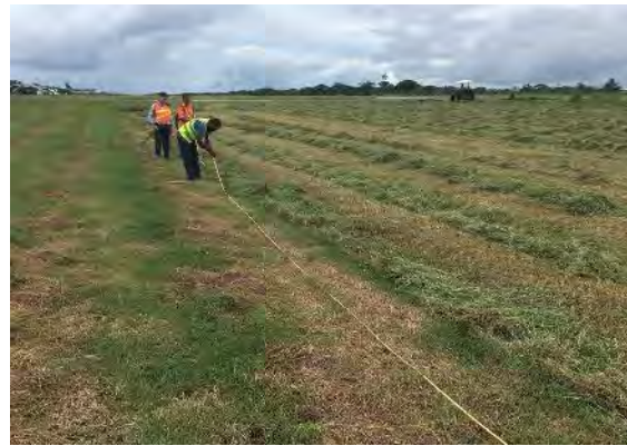
Photograph 10 Apron Expansion Area
