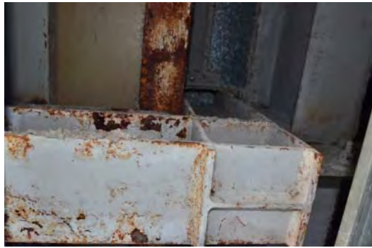
Photo 26 Back side of Ceiling at Airside
