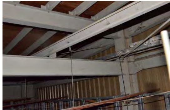
Photo 23 Condition of Structure of backside of the Ceiling (2)
