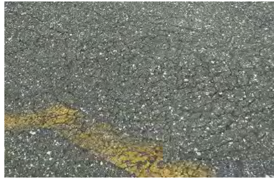
Photograph 8 Pavement on International Apron
