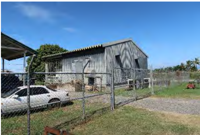
Photo 54 Existing Sub Station
