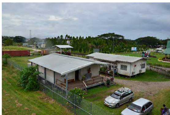
Photo 71 A Prefabricated Hut within the Terminal Area
