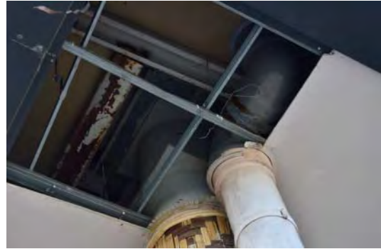
Photo 27 Back side of Ceiling at Airside
