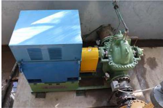
Figure 3-4 Installed Pump
