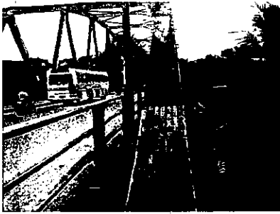
Loss of section of steel members due to corrosion
