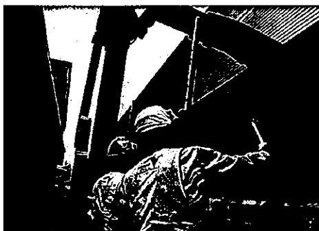
Hammering Inspection
