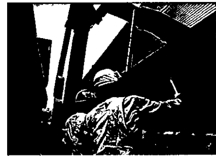
Hammering inspection by BIV
