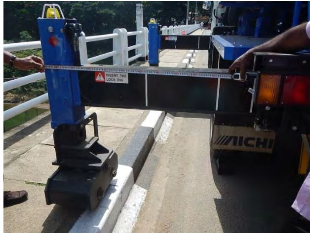
Photo 5.1 Example to position of the roller jacks on the service duct.
