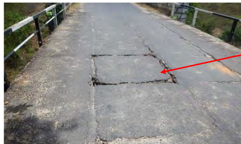
Photo 1.2 Unsupported RC Deck Slab
