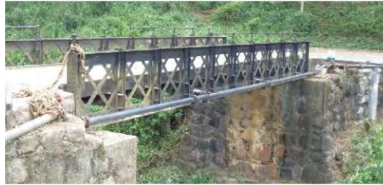
Photo 2.1 Half –through Bridge
