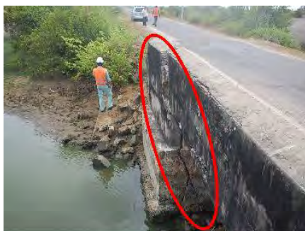
Figure 1 Example of Damage of Wing Wall
