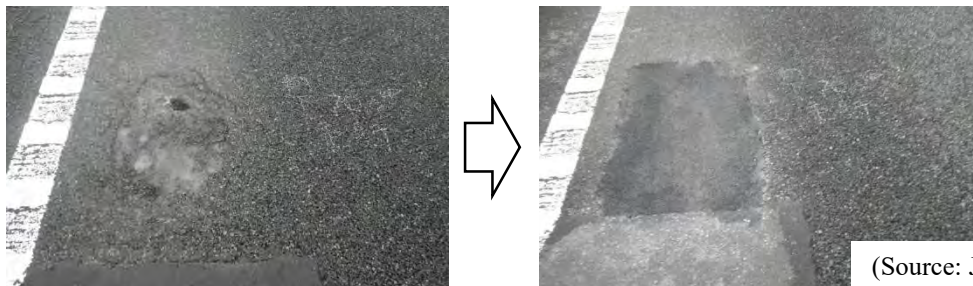
Filling of pavement mixture
