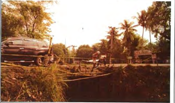
2016/10/21 Bridge inspection (Central Province)
