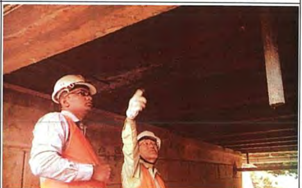
2016/8/10 Bridge inspection (Central Province)
