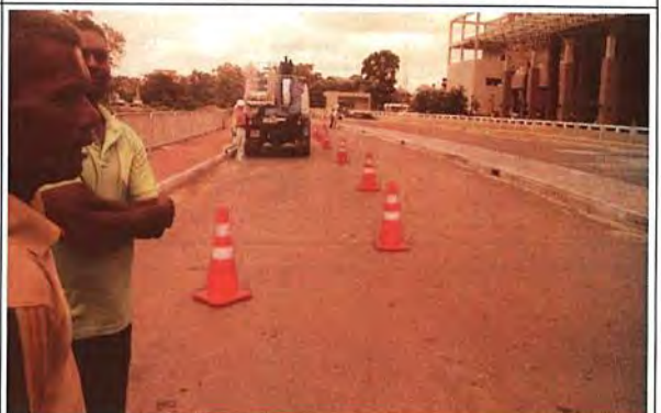
2017/5/30 OJT of traffic control for using BIV
