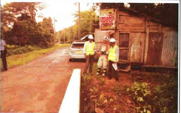
2016/11/23 Bridge inspection (Western Province)
