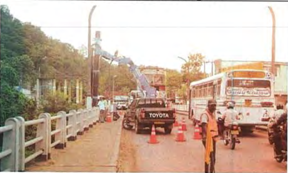
2017/6/13 Bridge inspection using BIV
