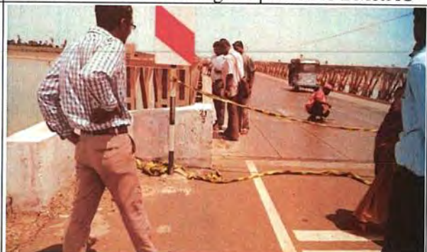
2015/10/13 Site investigation of repair work (Jaffna)
