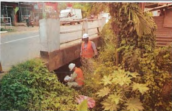
2016/8/5 Bridge inspection (Southern Province)
