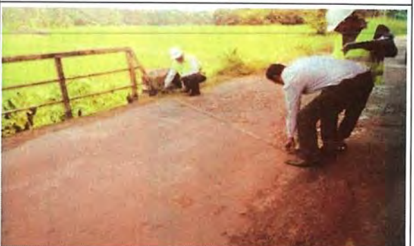
2015/12/9 OJT for bridge inspection
