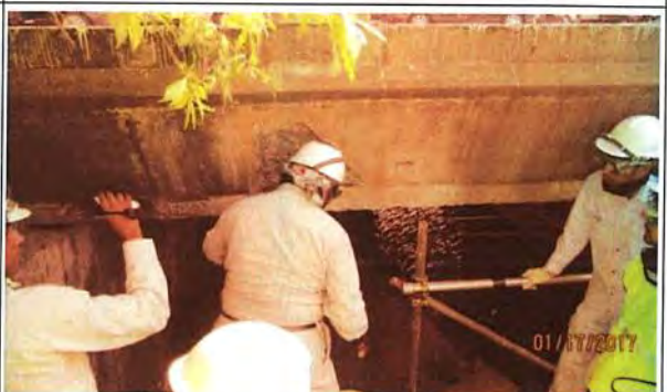
2017/1/17 Demonstration for plastering method
