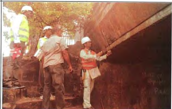
2015/9/15 OJT for bridge inspection to BM&AU
