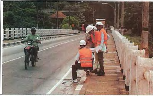
2015/7/8-10 Site investigation (Central Province)
