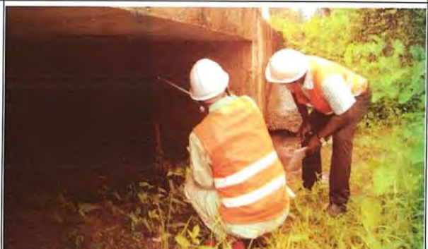
2016/7/27 Bridge inspection (Western Province)
