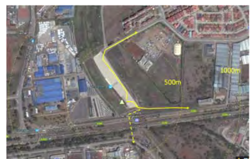
Fig. State of Practice, P&R facility in Imara Daima Sta.
