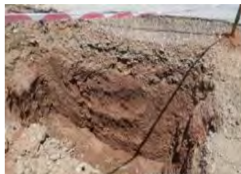
Trial pit near KP313 (near the end point)
