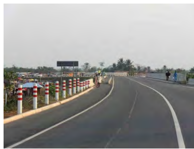
Example of combination of sign and protective wall
