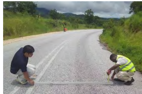
Photo 2 Road flatness check
