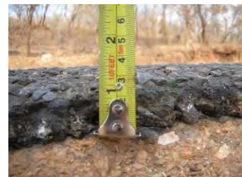
Existing Pavement Surface (thickness 3.5cm)
