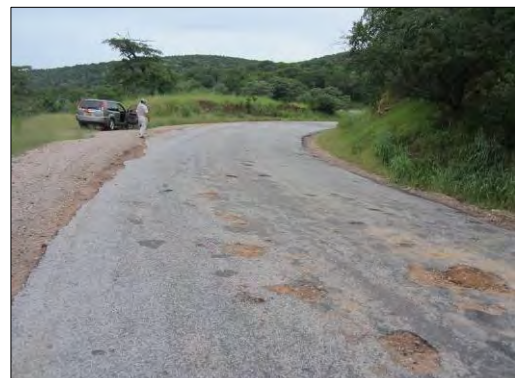
Photo 4 Road state at the 2nd field survey (February 2017, rainy season)
