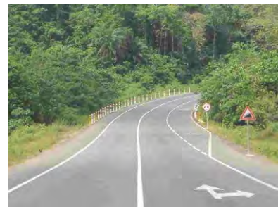
Example of forked part of hill climbing lane
