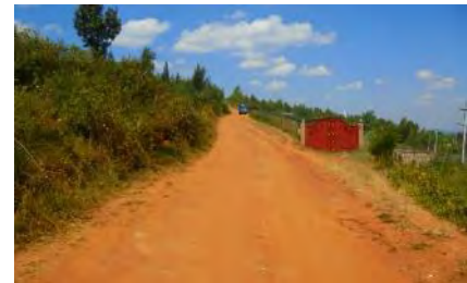
Fig. 2-2-1-4.2 Condition of the access road to Gasogi Substation
