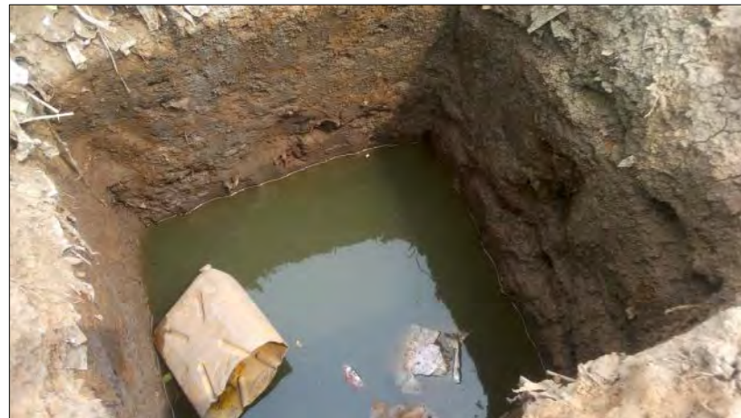
EXCAVATION ( test pit )
