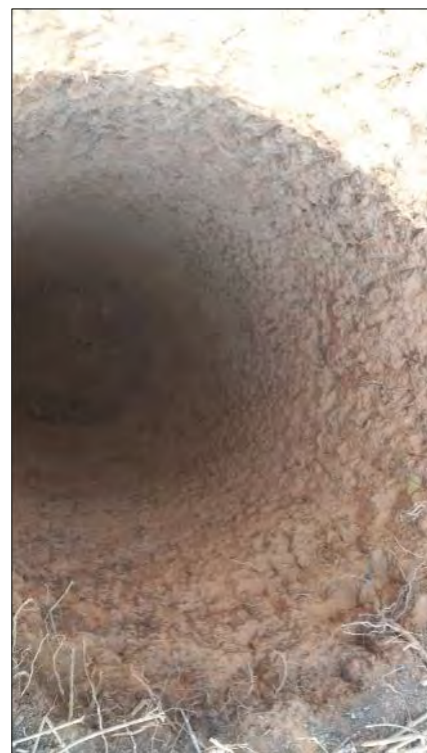
EXCAVATION ( test pit )
