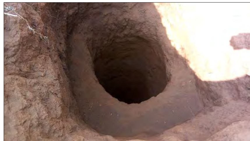
EXCAVATION ( test pit )
