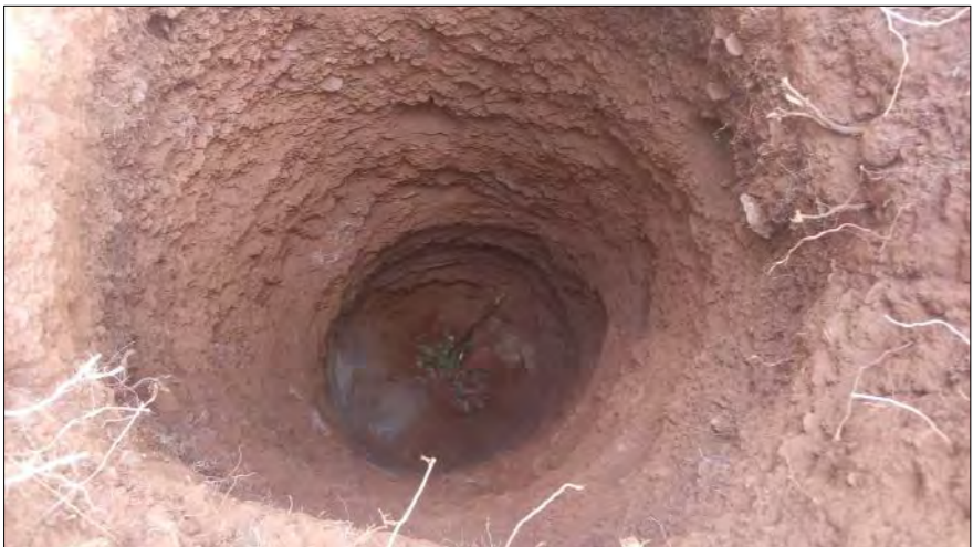
EXCAVATION ( test pit )
