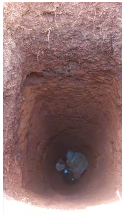
EXCAVATION ( test pit )
