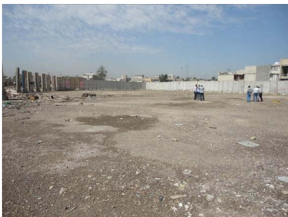
T-walls surrounding the Site
