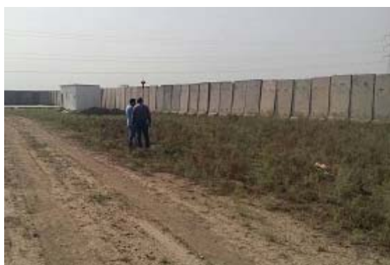
T-walls surrounding the Site
