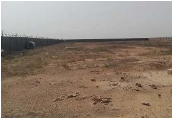
Walls surrounding the Site
