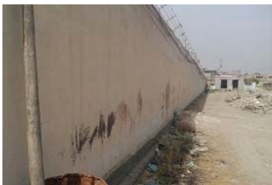
Walls surrounding the Site
