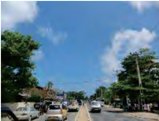
View at Pelawatta Road
