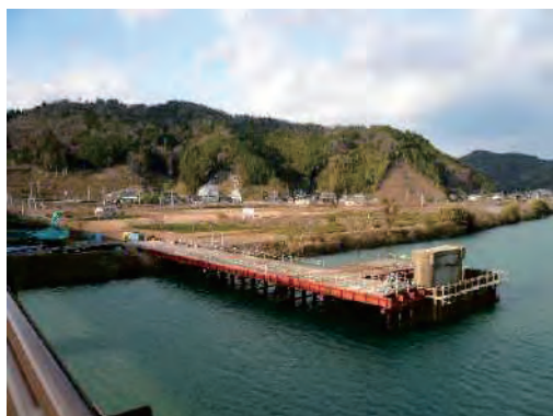
Figure 2.22 Sample Photos of Temporary Jetty and Cofferdam
