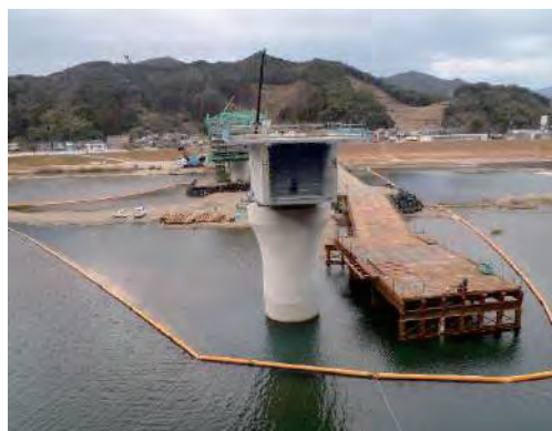
Figure 2.22 Sample Photos of Temporary Jetty and Cofferdam
