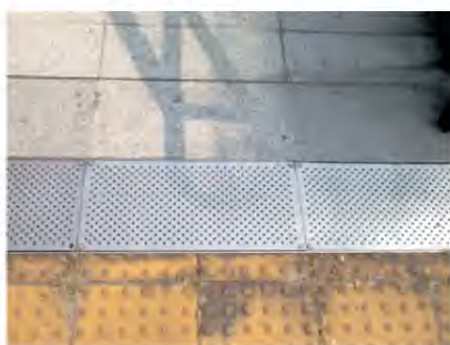
This drainage system is used in Thailand at the bottom of steps and ramps, and on the landings of ramps. It lies flat with the ground and the holes are not too big to catch mobility devices.
