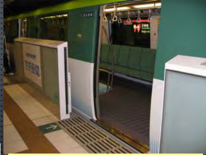
5mm gap height is realized. (in Fukuoka city subway)
