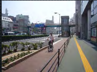
Elevator for a pedestrian deck
