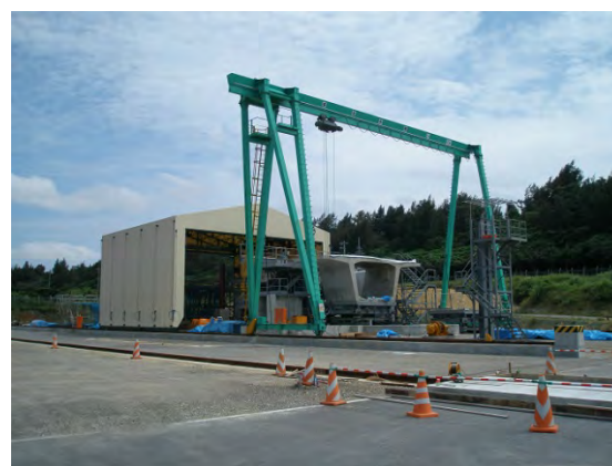
Figure 4.12.6 PC Box Girder Segment Manufacturing (Sample)
