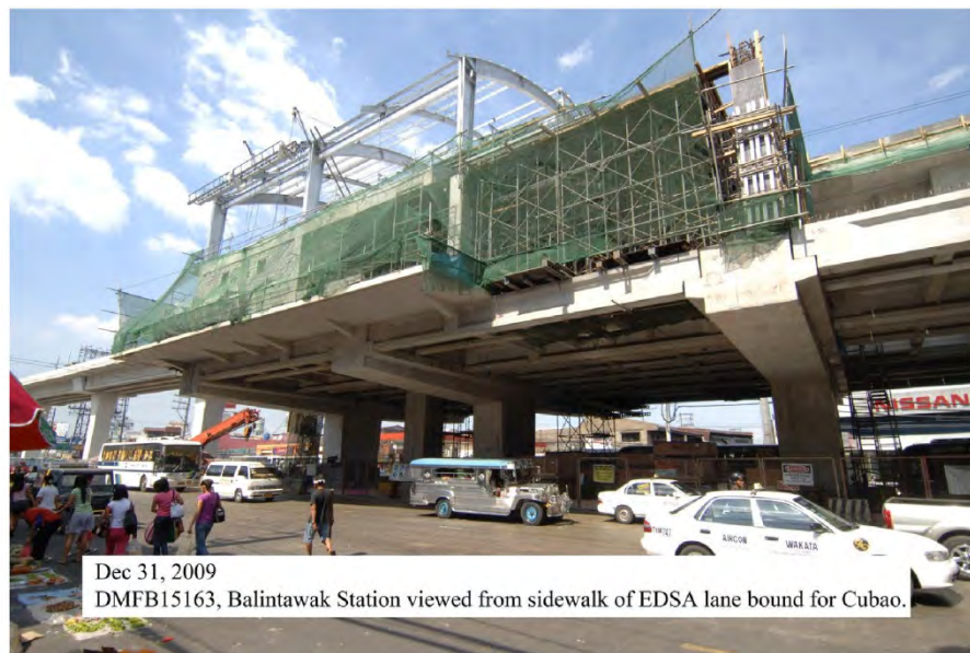
Figure 4.12.12 Station Platforms and Roof Frame under Construction (Sample)
