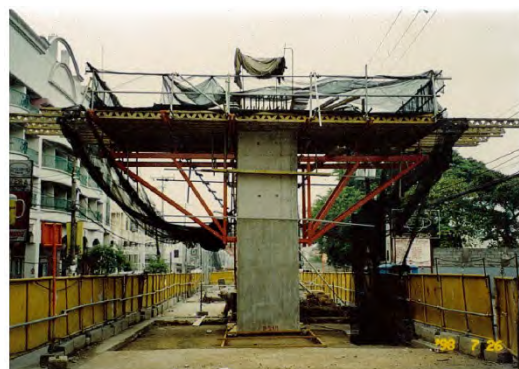
Figure 4.12.4 RC Pier Column Construction (Sample)
