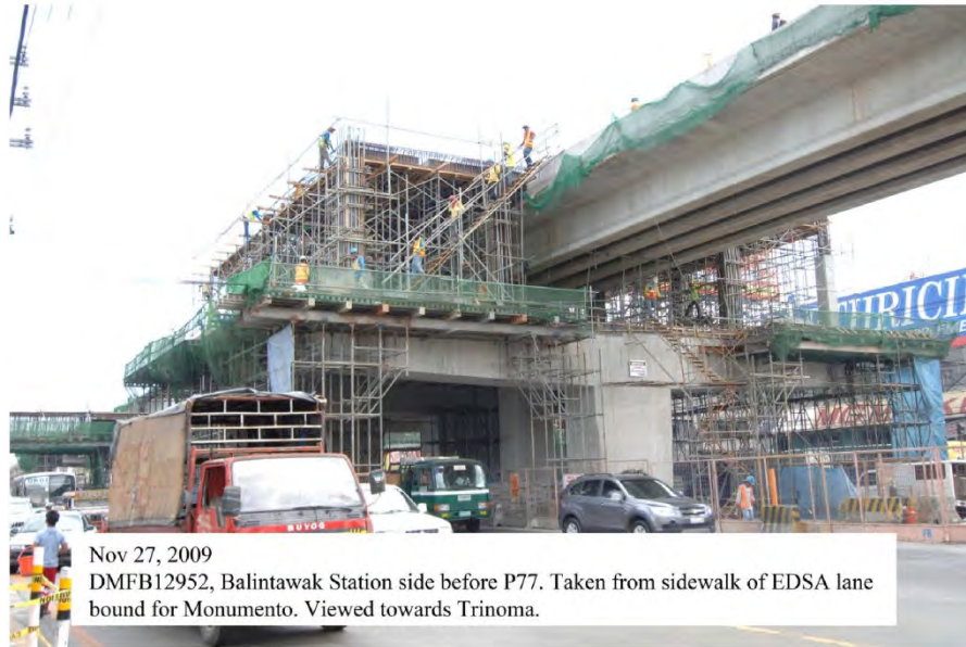
Figure 4.12.11 Station Concourse and Platform Construction (Sample)
