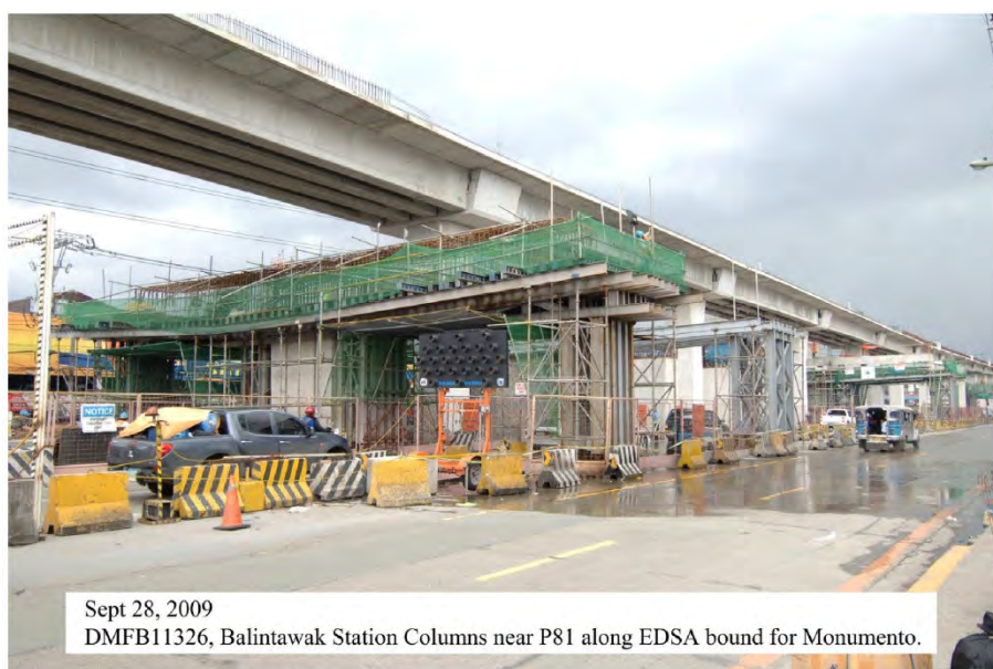
Figure 4.12.10 Station Cantilever Pier Construction (Sample)
