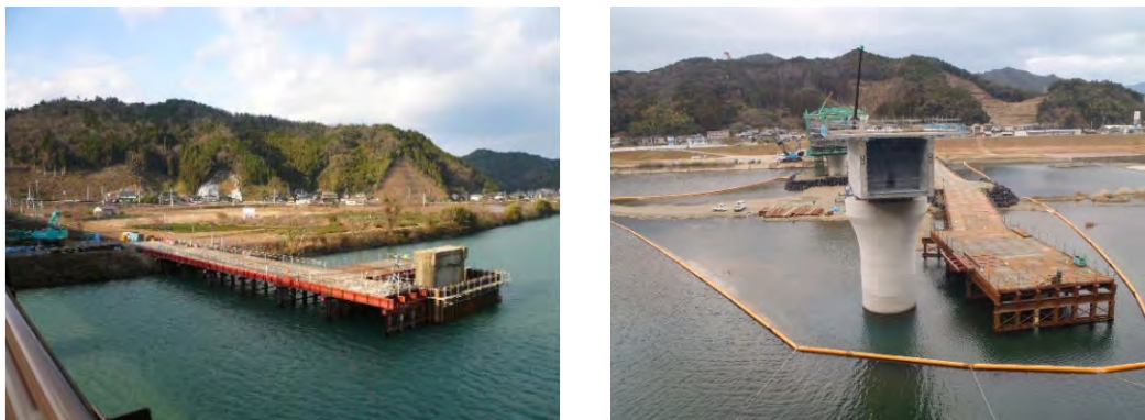
Figure 4.12.8 Temporary Jetty and Cofferdam (Sample)
