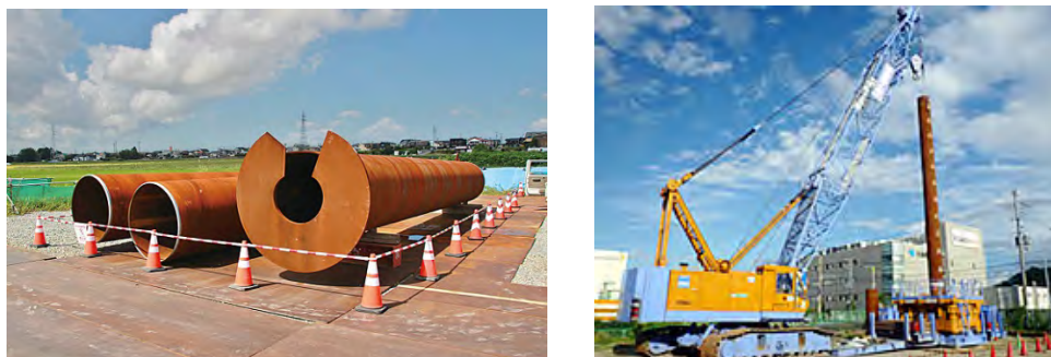
Figure 4.12.2 Screwed Steel Pile
