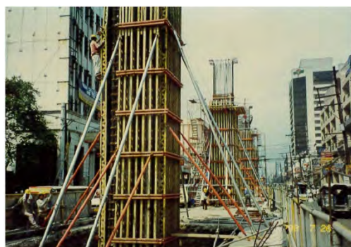
Figure 4.12.4 RC Pier Column Construction (Sample)
