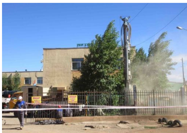
Photo 1 Drilling on the site
