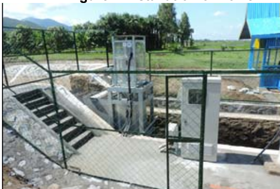
Figure-5 Installation of Power Archimedes – Standing Type (No.7 Drop)
