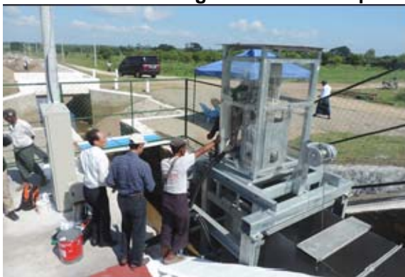
Figure-4 Installation of Power Archimedes - Hanging Type (No.3 Drop)
