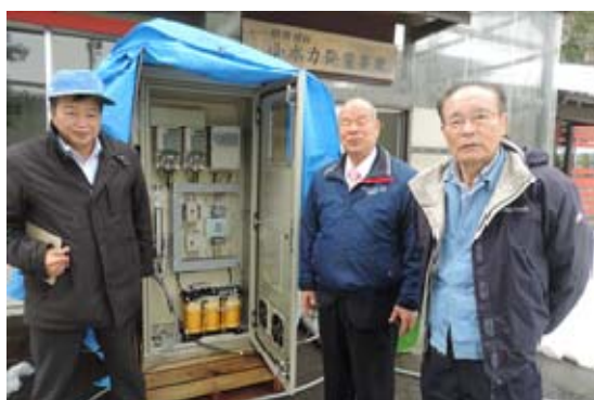
Inspection before Shipment
