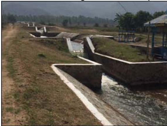
Figure-3 No.7 Drop/Fall of CY-3C Secondary Channel
