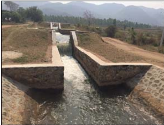
Figure-2 No.3 Drop/Fall of CY-3C Secondary Channel
