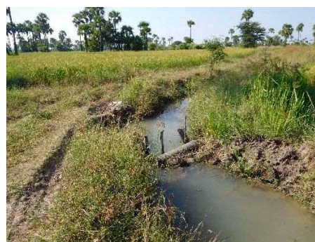
Local Check Structure in a Farm Ditch to Control Water by Sandbags
