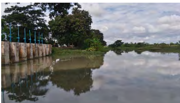
Spill-out with gate
