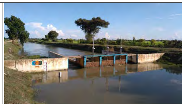
Cross Regulator (concrete structure type)
