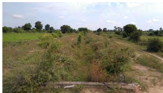
At D/S of Ayadaw Extension canal: Trees and weeds are growing in the canal due to no supply of irrigation water
