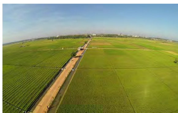
Example of land consolidation implemented in Nay Pyi Taw area (farm road and tertiary canals constructed)
