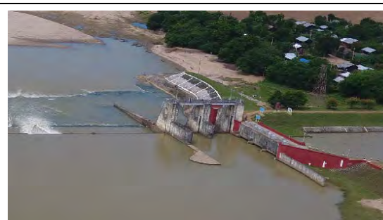
Head Regulator for YMC, Undersluice
