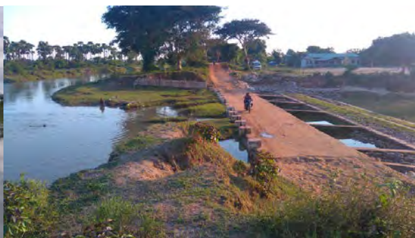
Overflow type Spill-out
