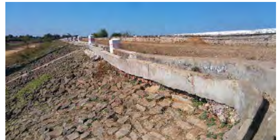
Condition of the downstream side of the dam body
