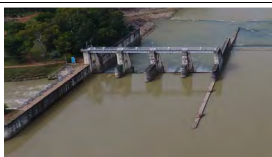
Head Regulator for SMC, Undersluice
