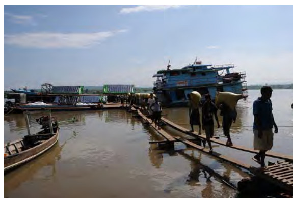
Kyauk Myaung Jetty: Left photo shows dry season condition, while right photo shows loading/ unloading condition during monsoon season. There is no concrete structure for this jetty, but only temporary installed wooden boards.
