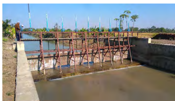
The structure (check structure) for the reuse of drainage water was constructed in drainage to supply the water to the land which is not irrigated enough and is not covered by irrigation system.
