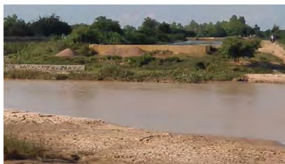
Sipadone (2) syphon: vibration occurs at around the inlet.
