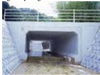
Figure 1.9 Image of Box culvert and bank protection
