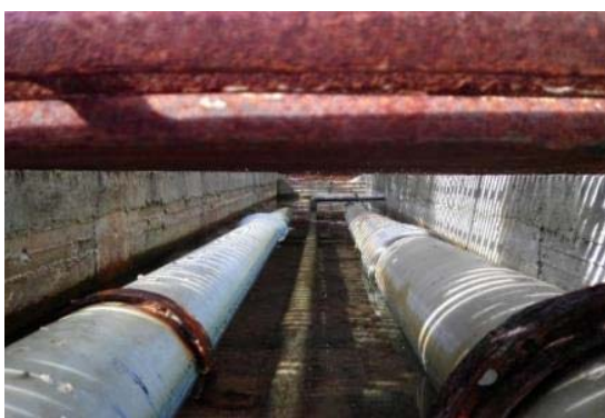
Existing and old intake pipe in pipe pit
