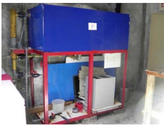
Tank P : Circulation system was taken out
