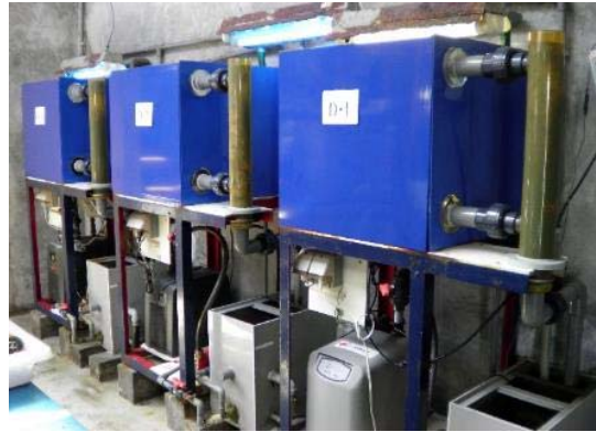
Tank D : Circulation system was aging
