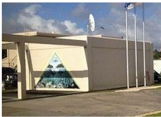
Exterior of Electric room
