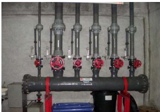
Header for branch pipes
