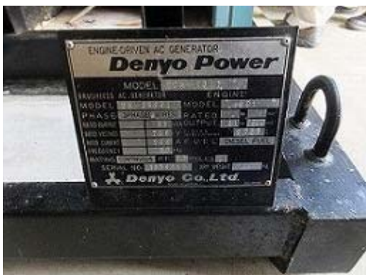
Nameplate of generator set
