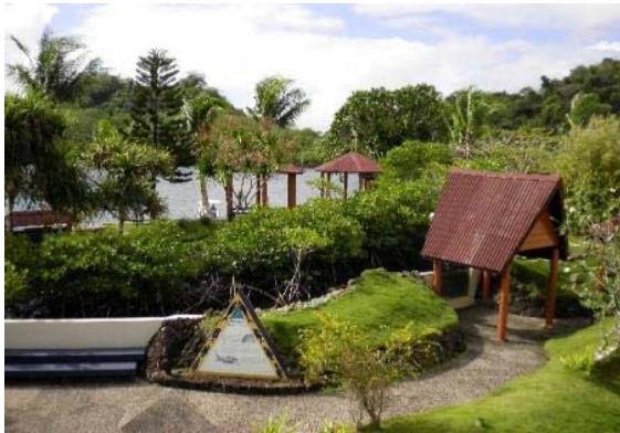
Outdoor tank J : Good condition
