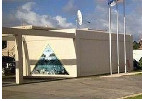
Exterior of Electric room
