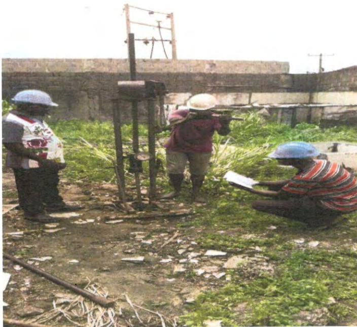
PICTURES SHOWING FIELD OPERATIONS ON THE PROJECT SITE
