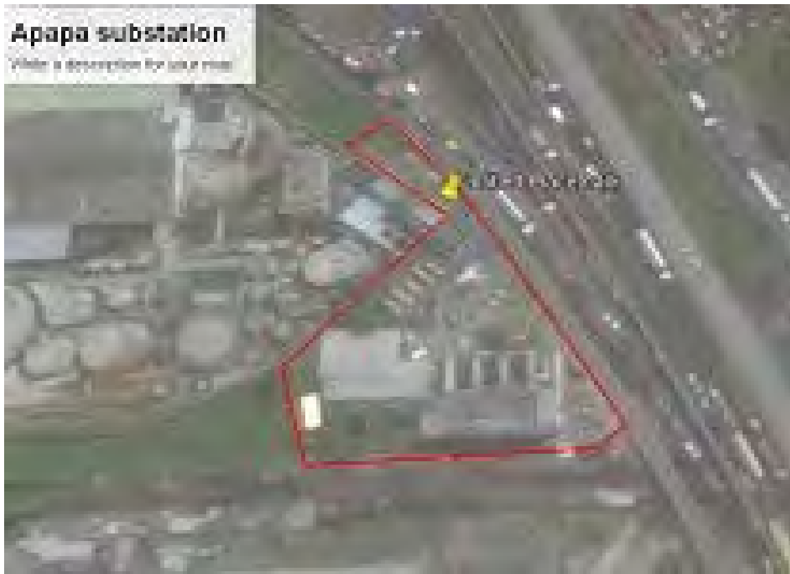
Figure 1: Enclosed Boundary of Apapa Road Substation
