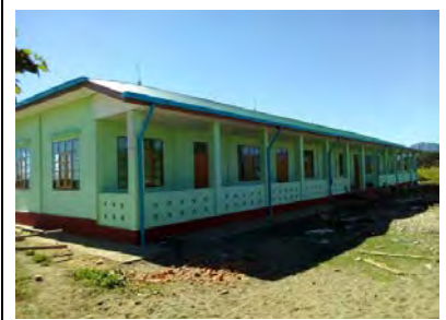
120'x30' RCC1 (6 Classrooms) November 2017
