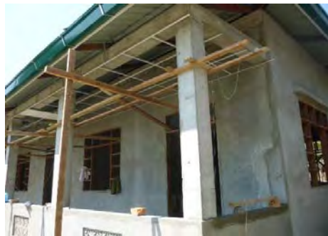
3-3c Scaffolding fixed to window/door frame by long nail
