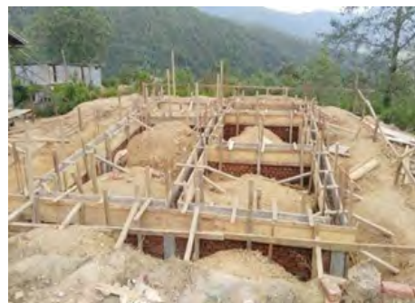
1-20 Formwork for plinth beam
