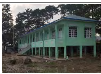
120'x30' RCC PL6' (6 Classrooms) August 2017
