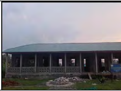
120'x30' RCC1 (6 Classrooms) September 2017
