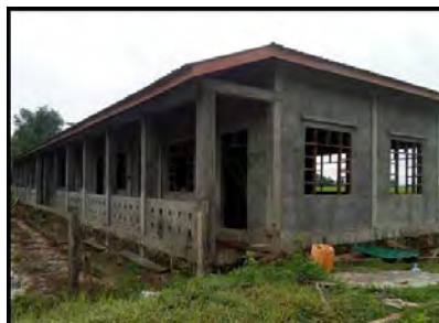
120'x30' RCC1 (6 Classrooms) September 2017
