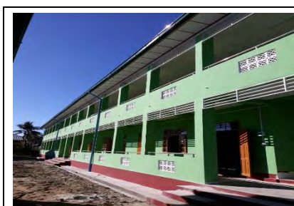
44'x30' RCC2 ( 8 Classrooms)-1 January 2018
