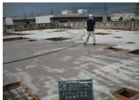
3-7 Curing after floor concrete
