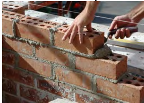
3-1 Fill mortar to brick joint without gap
