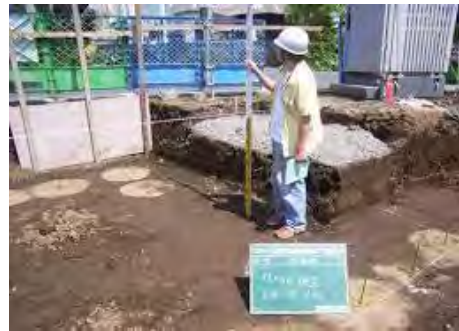
1-5 Check excavated level
