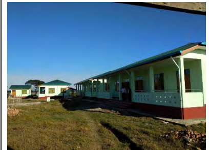
60'x30' RCC1 (3 Classrooms)-1 March 2018
