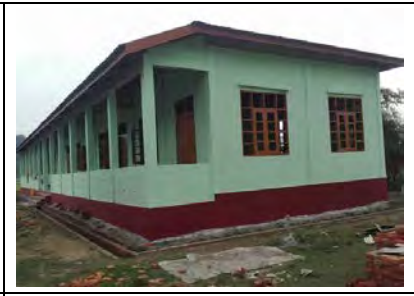
120'x30' RCC1 (6 Classrooms) November 2017
