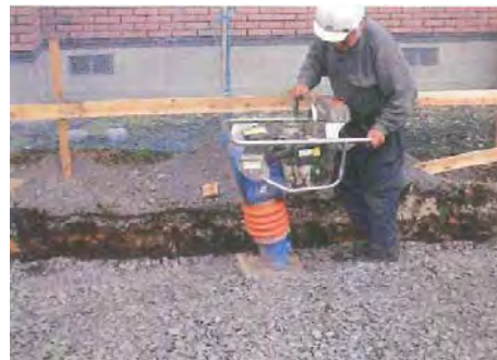
1-6 Compaction of hardcore by rammer
