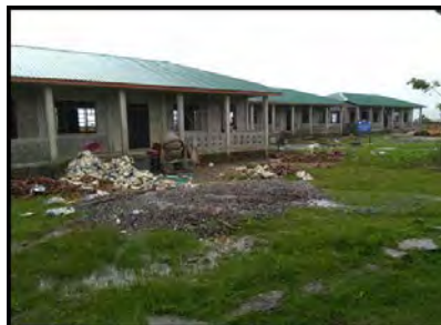
60'x30' RCC1 (3 Classrooms)-1 September 2017
