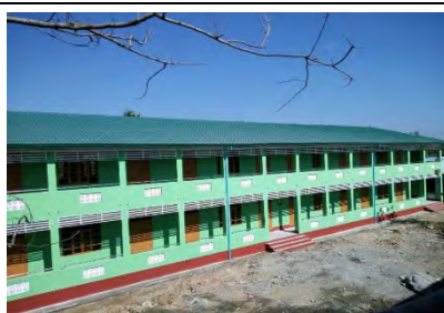
144'x30' RCC2 ( 8 Classrooms)-2 January 2018
