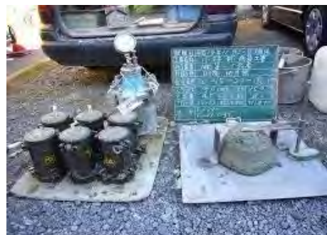
1-10a Fresh concrete test
