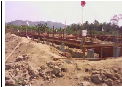
120'x30' RCC1 (6 Classrooms) February 2017
