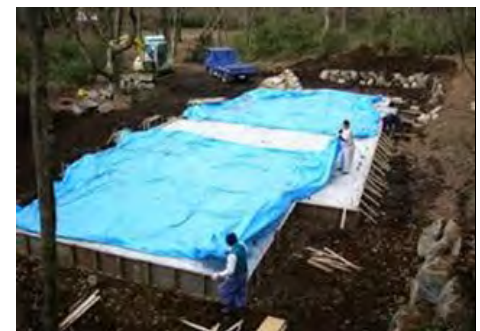
1-10c Concrete curing by plastic sheet
