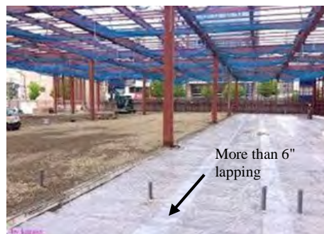
3-6 Polyethylene sheet (0.15mm thk.) laying
