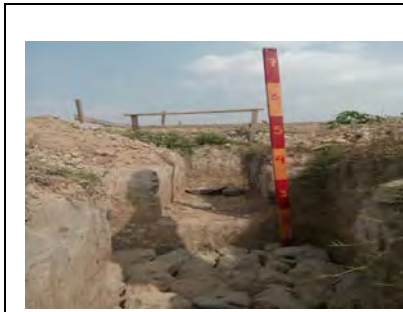
60'x30' RCC1 (3 Classrooms)-1 February 2017
