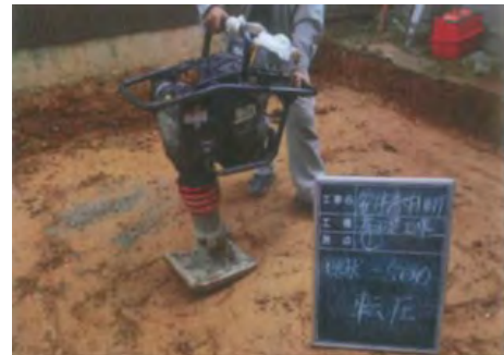
1-18 Compaction during backfilling
