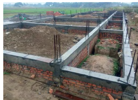
1-21 Concrete pouring for plinth beam has been completed
