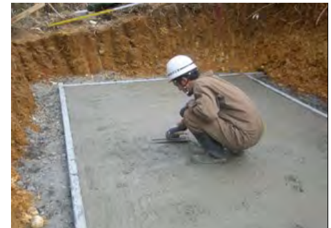
1-7 Lean concrete pouring
