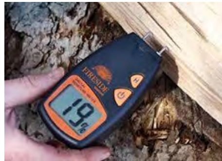
3-3a Check water content before installation
