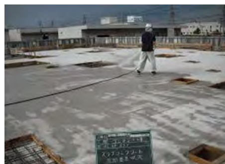
3-7 Curing after floor concrete
