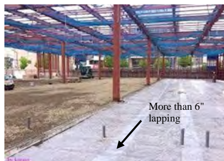
3-6 Polyethylene sheet (0.15mm thk.) laying
