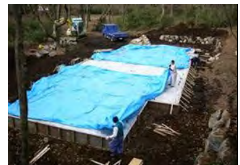
1-10c Concrete curing by plastic sheet
