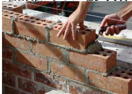
3-1 Fill mortar to brick joint without gap
