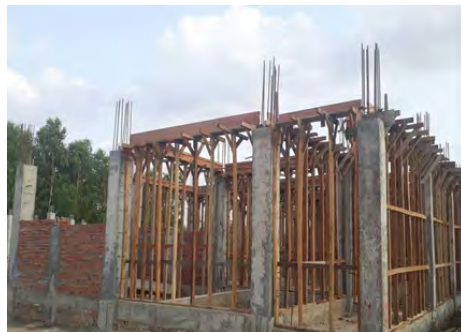
2-4 Form and prop of beam form
