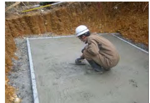
1-7 Lean concrete pouring
