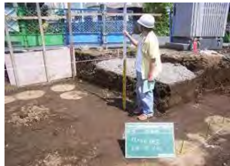
1-5 Check excavated level
