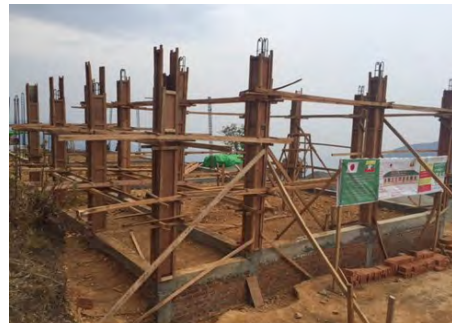
2-2 Formwork for column
