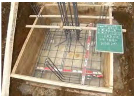
1-8,9 Formwork and rebar placing for footing
