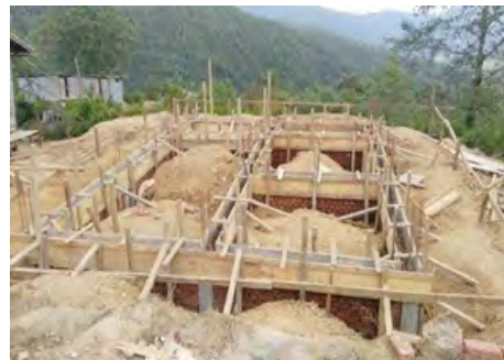
1-20 Formwork for plinth beam
