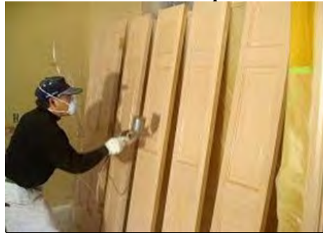
4-7b Door painting before installation
