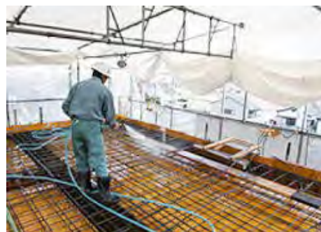
2-6b Water spreading before concrete pouring
