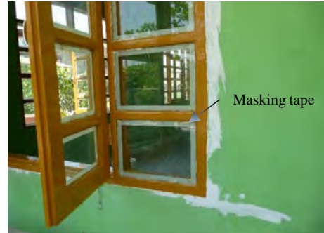
4-9 If install glass before painting, glass protection is necessary
