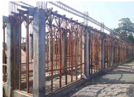
2-5a Placing of beam rebar
