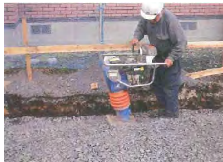
1-6 Compaction of hardcore by rammer
