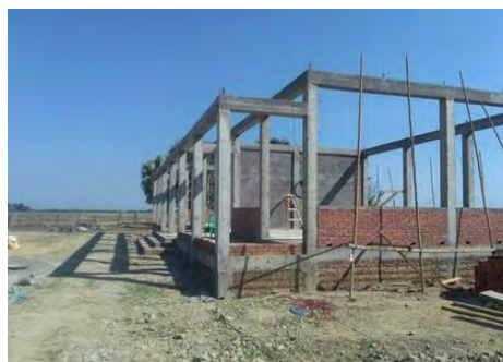
2-6a Concrete pouring for beam has been completed
