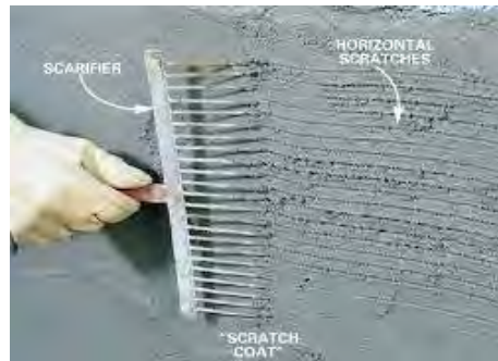
3-4a Scratch coat of wall plaster mortar mix Cement:Sand=1:3
