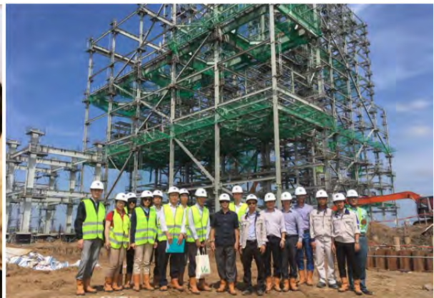
【Site visit with Counterpart, 9 December 2016】
