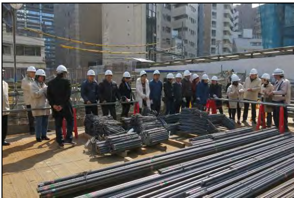
Site visit (S3) / 28 Feb. 2018 Complex Building (Construction Site) (Minato Ward, Tokyo) Government Building Planning Division Kanto Regional Development Bureau, MLIT
