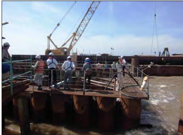
(b) Lach Huyen Port (Road and Bridge)
