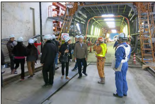
Site visit (S3) / 10 Nov. 2016 Tokyo-Port Tunnel (Construction Site) (Shinagawa Ward, Tokyo) Kawasaki Road Office Kanto Regional Development Bureau, MLIT
