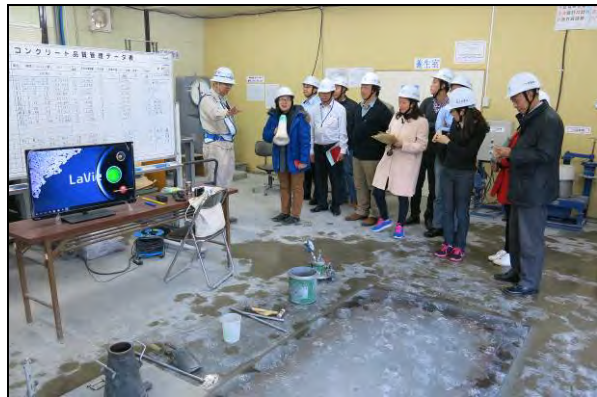
Site visit (S2) / 15 Nov. 2016 Yamba Dam (Construction Site) (Naganohara Town, Gunma Pref.) Yamba Dam Work Office Kanto Regional Development Bureau, MLIT
