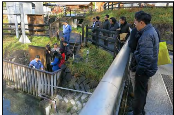
Site visit (S8) / 15 Nov. 2015 Neutralization Facility for strong acid river water (Kusatsu Town, Gunma Pref.) Sinaki Dam Water Control Office Kanto Regional Development Bureau, MLIT
