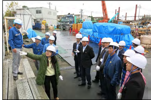
Site visit (S5) / 20 Nov. 2015 Oowada Pump Station (Ichikawa City, Chiba Pref.) Japan Sewage Works Agency, Kanto and Hokuriku General Office
