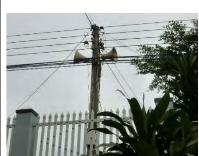
Fig 6. Loudspeaker used for flood warning
