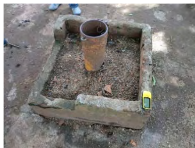
Fig 5. Dried up deep well (D=150 mm). In 2004 it was drilled by 95 m depth but water did not come out.
