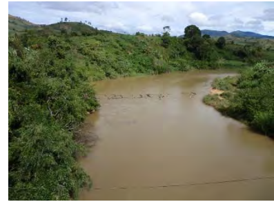
Fig 9. Destroyed bridge due to flooding
