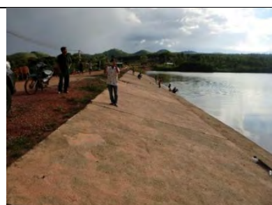
Fig 1. Dak Mhang reservoir (earth fill dam, capacity=0.657 MCM) operated by IMC and constructed in 1984. In 2015/16 drought, this reservoir was dried up.
