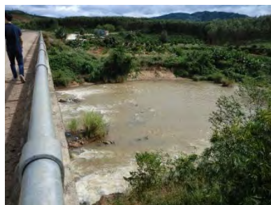
Fig 7. Dak Pxi river telemetric river water level gauge installed place (light bank)
