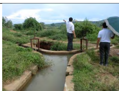
Fig 2. Irrigation canal from Dak Mhang reservoir (Q=0.37 m 3 /s) operated by IMC.
