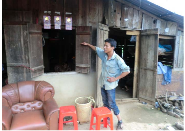
Victim showed the flood water level in 12/2016 (District: Di Linh, Commune: Tam Bo)
