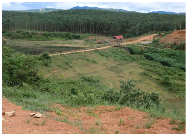
Dak Trit Irrigation Reservoir (District: Dak Ha, Commune: Dak La)
