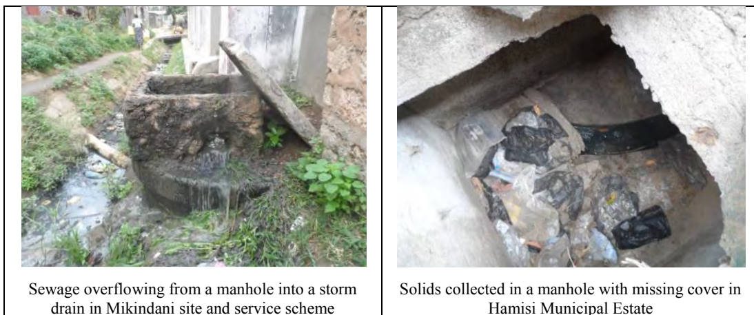
Figure 5.2.3: Existing Sewer Pipe and Manhole
