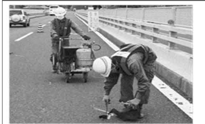
Photo Injection of an Asphalt-Type Sealing Material
