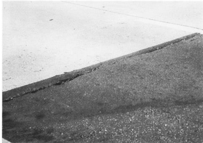
Figure 5.6.4 Roughness due to structure buried under the ground
