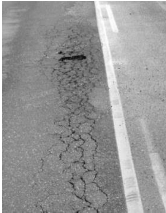
Image 5.5.12 Alligator cracks
