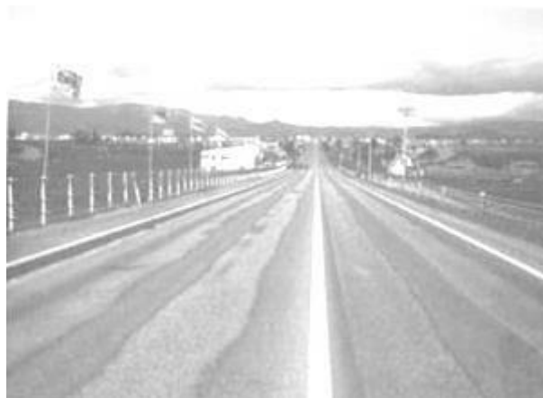
Image 5.5.14 Rutting caused by asphalt deformation
