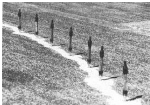
Image 5.6.13 Injection by pressure of rubber tube
