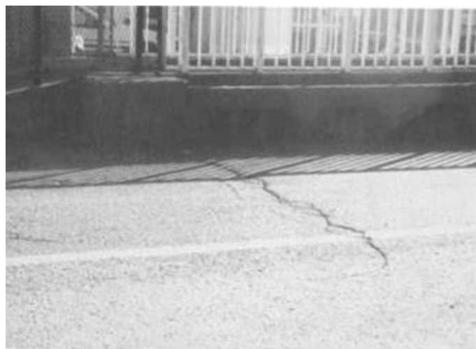
Image 5.5.13 Grade Depression at Structures
