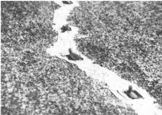
Image 5.6.13 Injection by pressure of rubber tube
