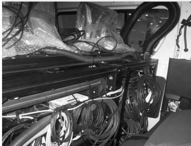
Figure 12.38 Sorting and fixing the cables to the rack
