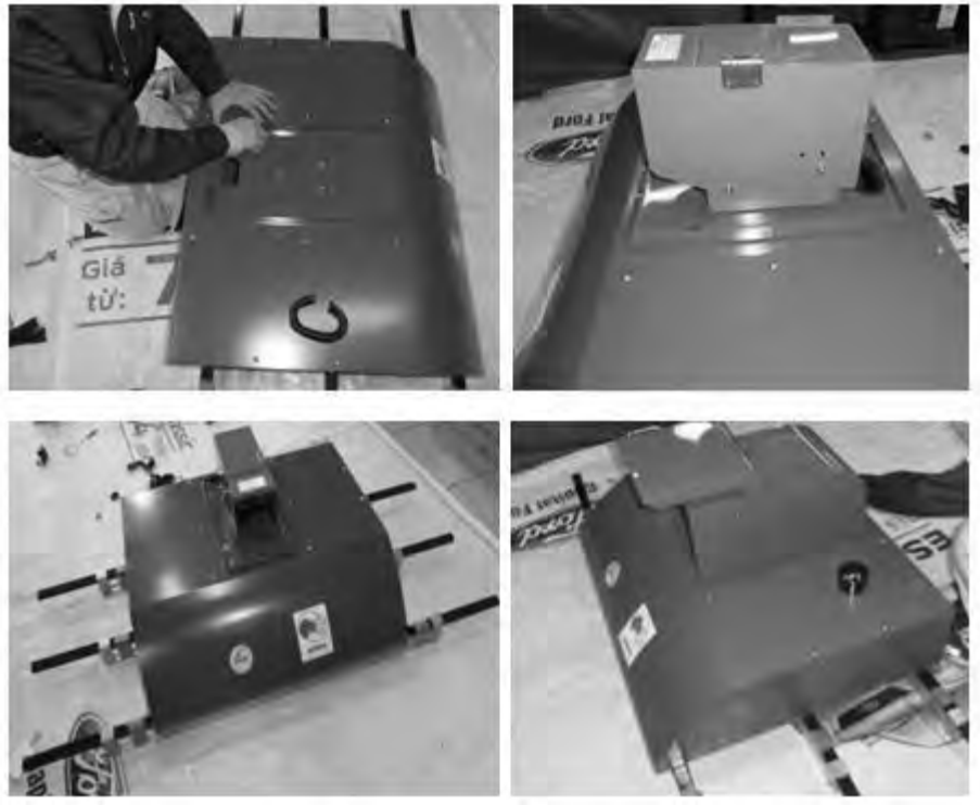
Figure 12.10 Attach the camera for front image on the front platform
