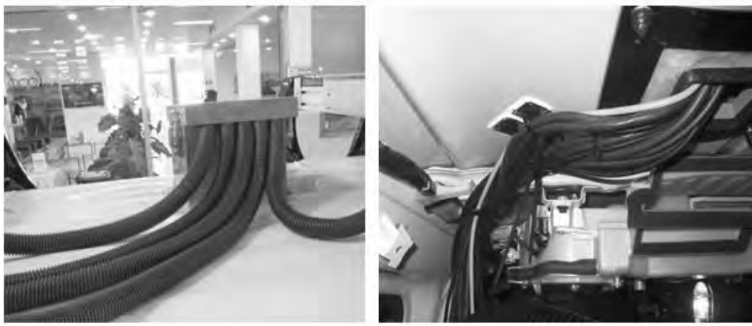
Figure 12.34 Wiring the cables from outside to inside of the car
