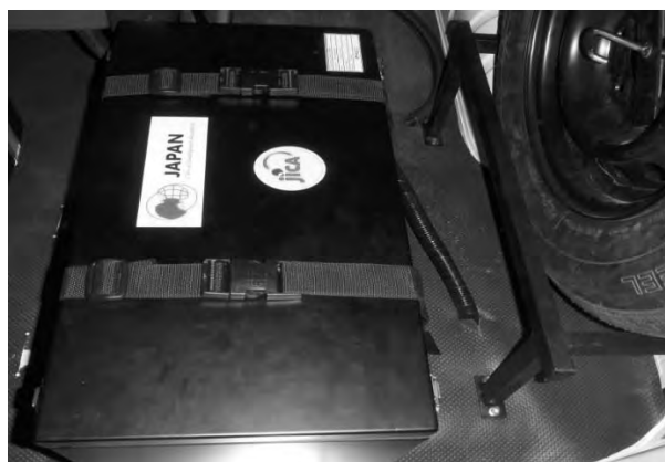
Figure 12.18 Fixing the case of sub battery on the floor
