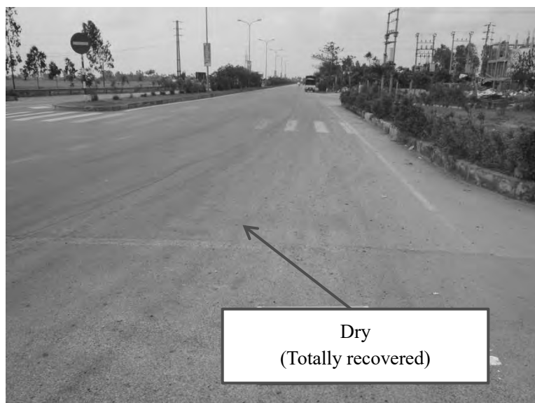
Figure 3.25 Road conditions where survey can be restarted (sample-2)
