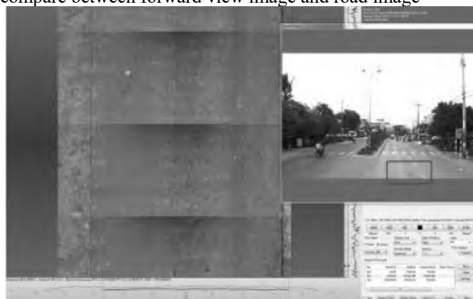
Figure 4.19 Example of visible the crack only forward view image
