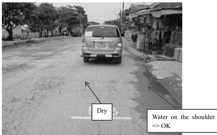
Figure 3.24 Road conditions where survey can be restarted (sample-1)
