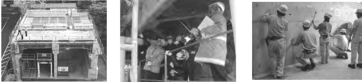
Figure A8.2.3 Image of N2U Bridge
