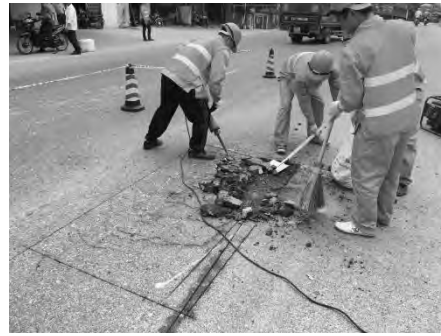
Remove existing surface
