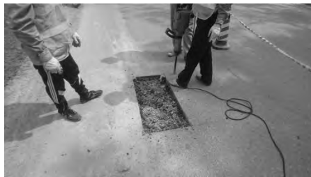
Remove existing Surface
