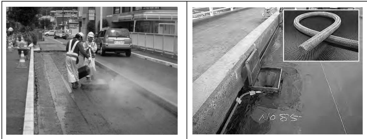
Photo 6.1-3 Pilot Repair Work (Bridge Waterproof)
