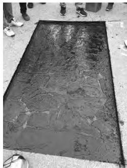
Prime coating on basement layer
