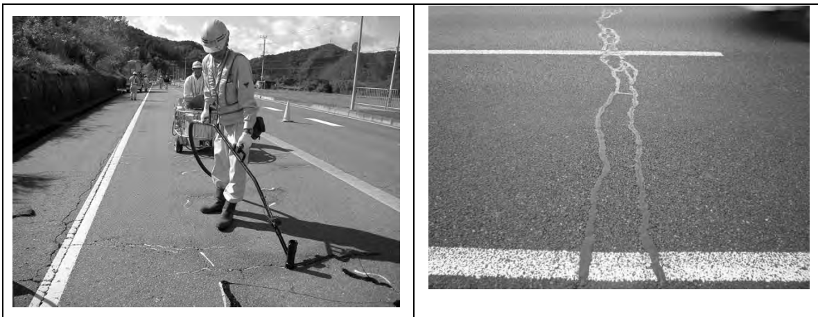
Photo 6.1-1 Pilot Repair Work (Crack Sealing)
