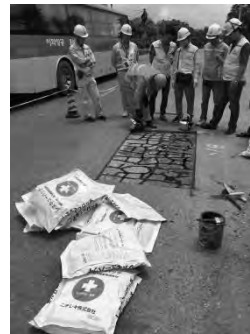
Mend of crack on top of basement layer
