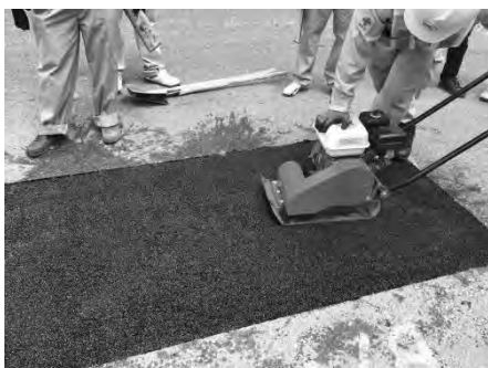
First layer compaction
