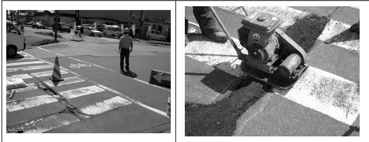
Photo 6.1-2 Pilot Repair Work (Patching)
