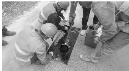
Prime coating on basement Layer
