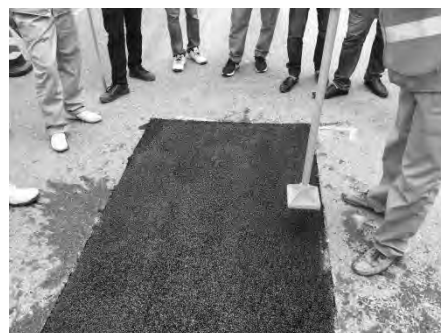
First layer compaction
