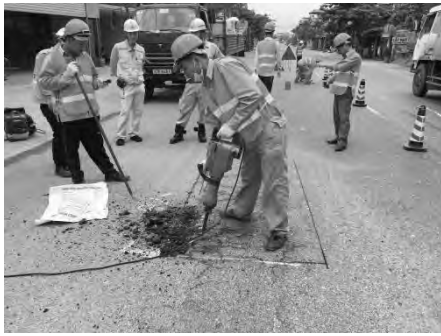
Remove existing surface
