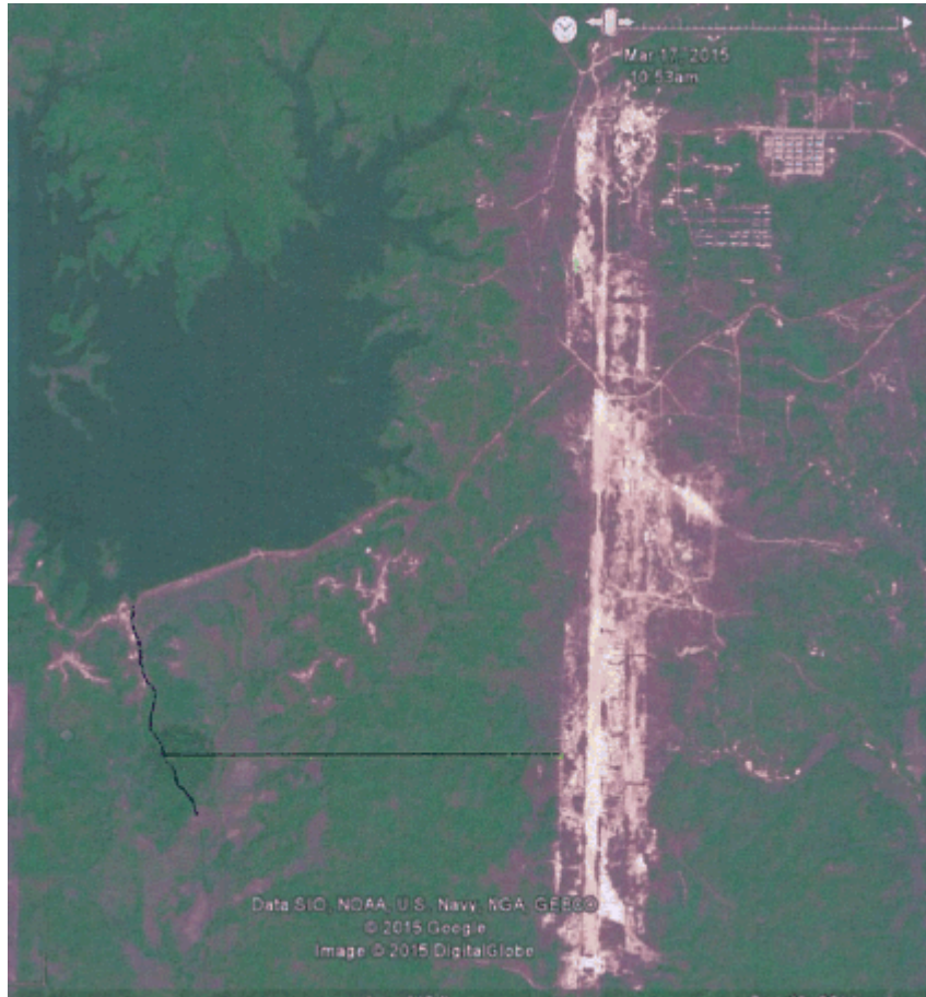
Figure 2.8.16 Location of Drainage Canal
