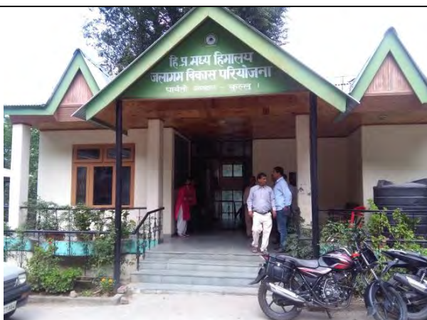
Proposed Regional Office for the Project, Kullu District (15 June 2017)
