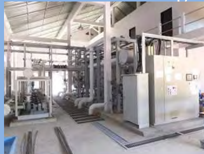
Water Purification System for Highiy Turbid Water =Fiber filters (Actifiber) and Sand filtration System.
