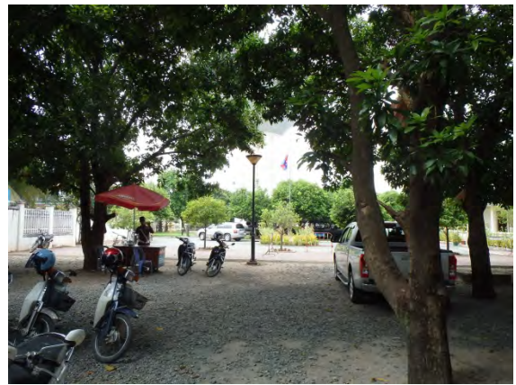
1-4: Planned construction site for the WTP (Nov. 2017)
