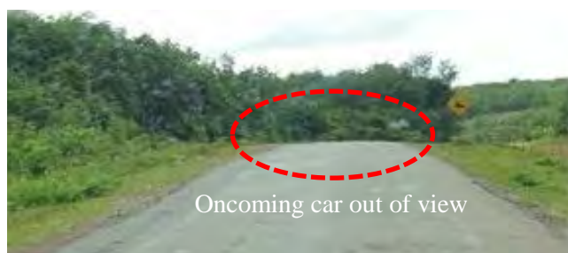
Figure-8.3.12 Substandard Vertical Alignment on NH-8
