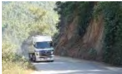
(Earth cutting slopes on the corridor)
