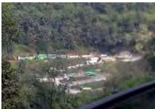
(Queuing heavy vehicles to pass the valley, Goat Twin Viaduct is proposed to cross the valley)
