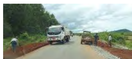
(widening to 2-lane by bituminous treatment)
