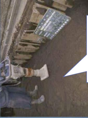
Using improved soil and adequate compaction
