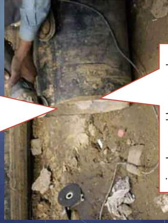
pipe has not been cut straight. No water leakage?
