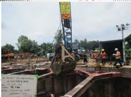
21. Laying Gravel Materials
