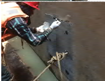
41. Mortar Filling Work & Curing
