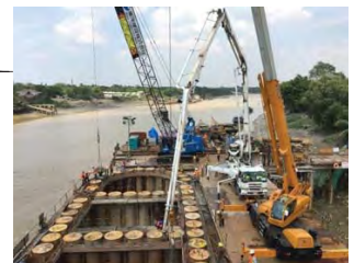
Concrete Filling inside SPSP (8000mm)
