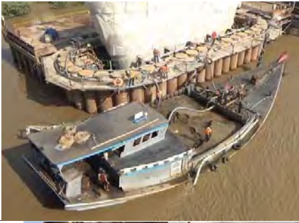
39. Backfilling inside the cofferdam
