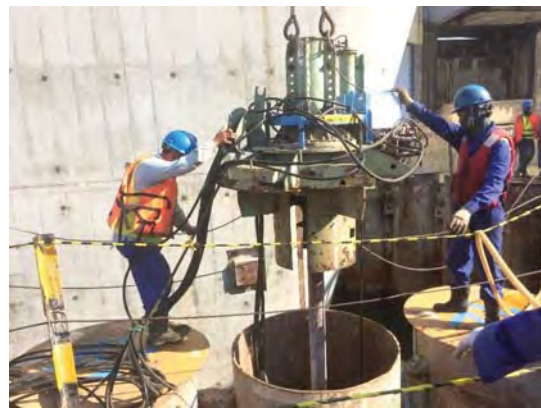
41~42. Cutting and Lifting of SPSP
