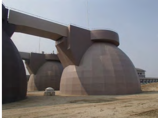
Sewage treatment tanks, Japan
