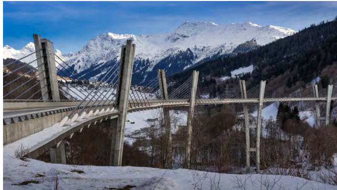
Sunniberg bridge, Switzerland
