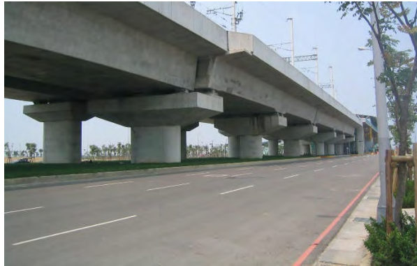
Taiwan High Speed Rail Viaduct (Chiayi Station), Taiwan
