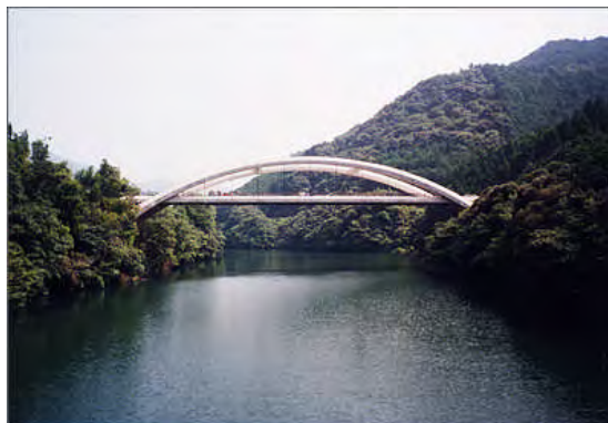
Miyagawa Bridge, Japan
