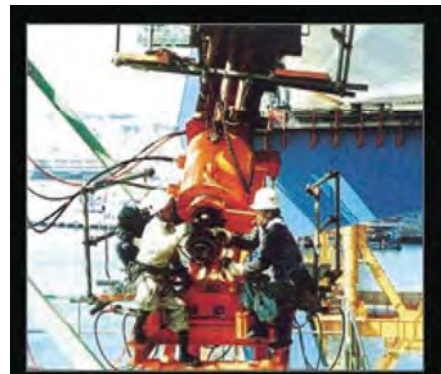
Cable tensioning
