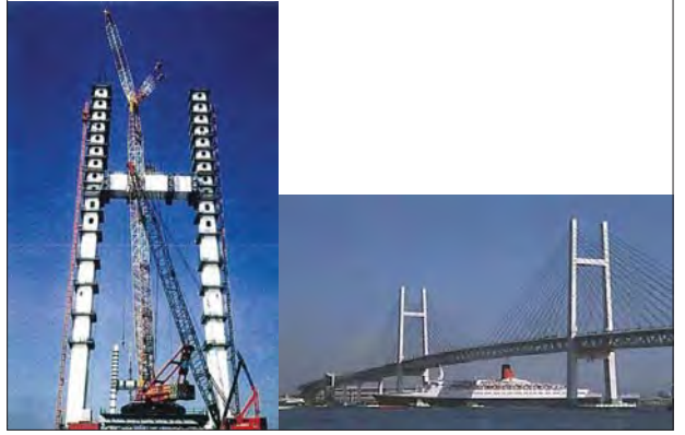
Crawler crane and tower crane
