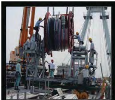
Reeled cable set to unreeler machine
