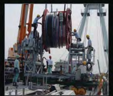
Reeled cable set to unreeler machine
