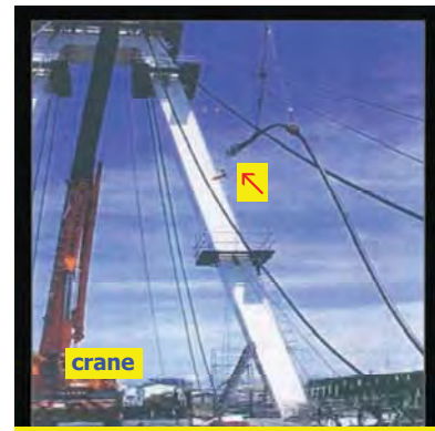
Lift up of cable socket to tower anchorage
